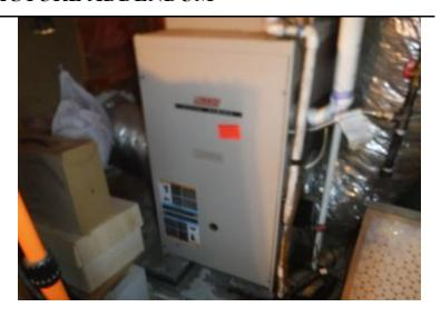
Standing water noted in the drain pan of the basement furnace. The furnace sump pump is not operating. Recommend having a licensed contractor replace the sump pump.
